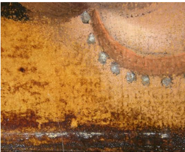
Figure 10: Detail showing frame abrasion, bottom centre.
